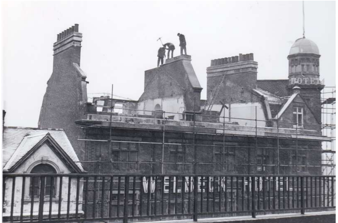
Working at Height on the Welbeck Hotel, Nottingham, 1970
